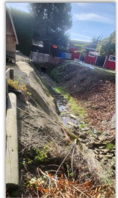
Open drainage behind Marianne's
