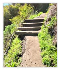
As you can see from this photo, the erosion further narrowed the trail and undercut the new staircase. Our approach to solving this issue is to engage the State Parks personnel to develop a repair strategy as we wait until the rainy season has ended. Stay tuned!
