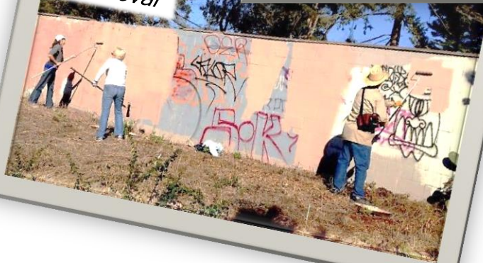
Rail Line Graffiti Removal
