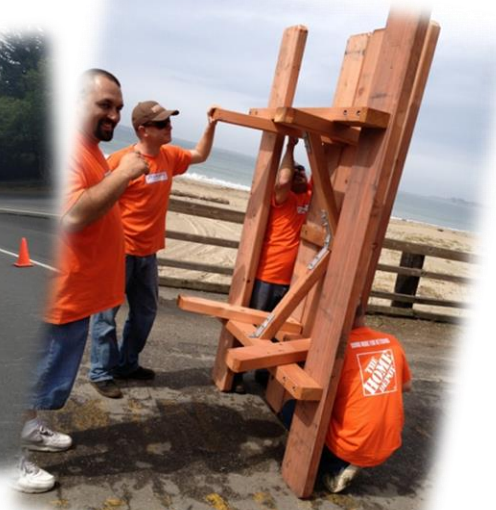
Building picnic tables
