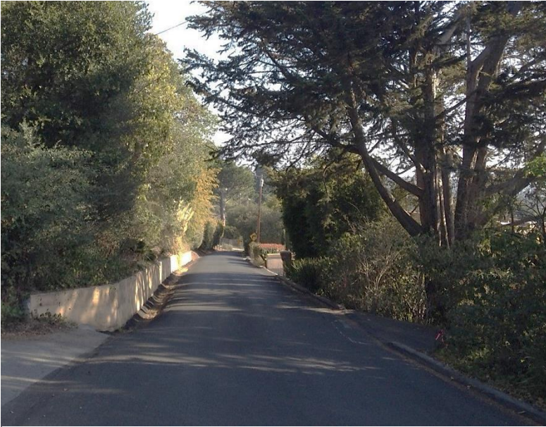
Neighbors up the hill on Viewpoint Road in Aptos formed a County Service Area and used their funds to repave the entire street.
